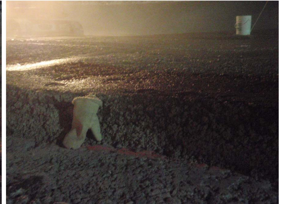
Photo 10: View of lift thickness placed today. Photo taken around station 0+85.
