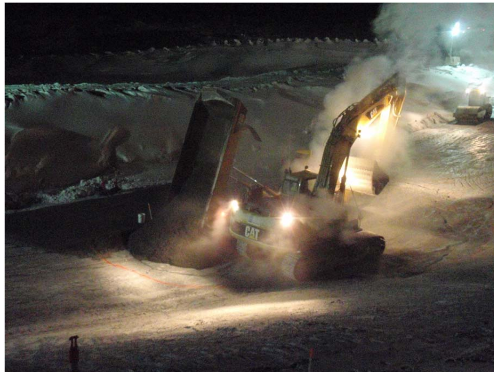
Photo 12: ~N view of FCM placement in the central key trench area.
