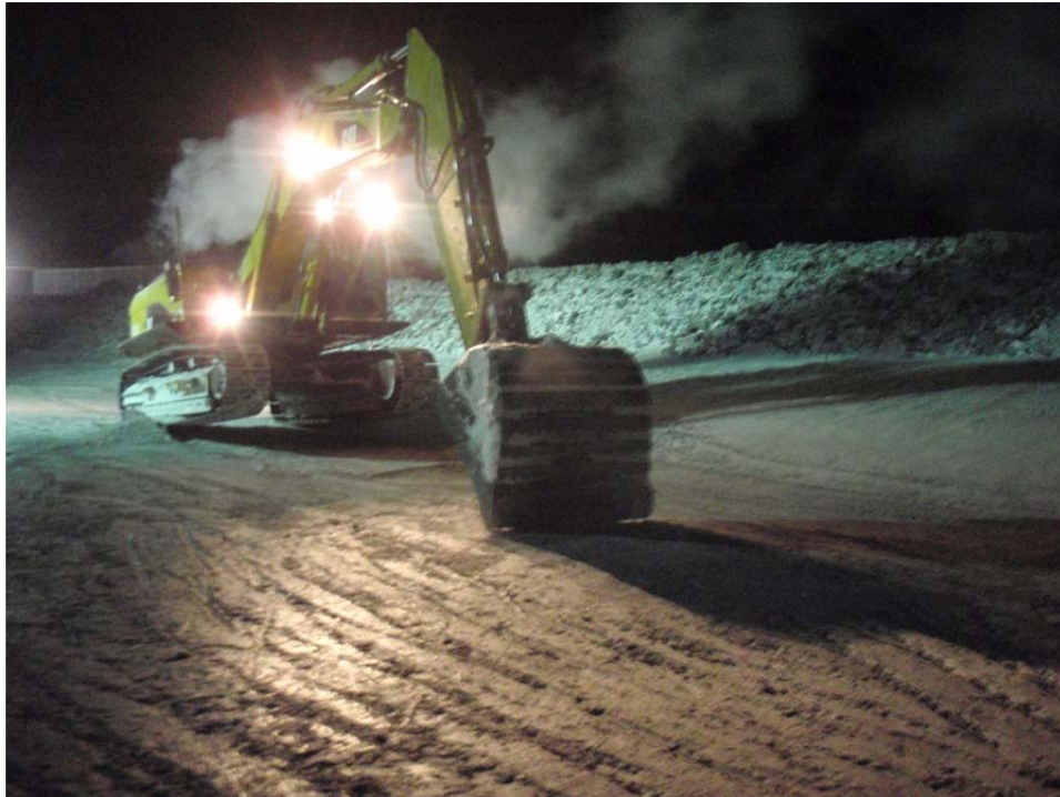
Photo 8: CAT 33 CL Excavator (equipped with finishing bucket) scraping down 5/8" material in the key trench. Note that the excavator is working around station 1+20 at the time this picture was taken.
