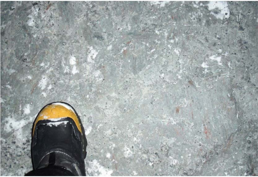
Photo 5: Close-up view of appearance of typical key trench base after most of 5/8" clear material has been removed, taken around station 1+00 before dental cleaning.
