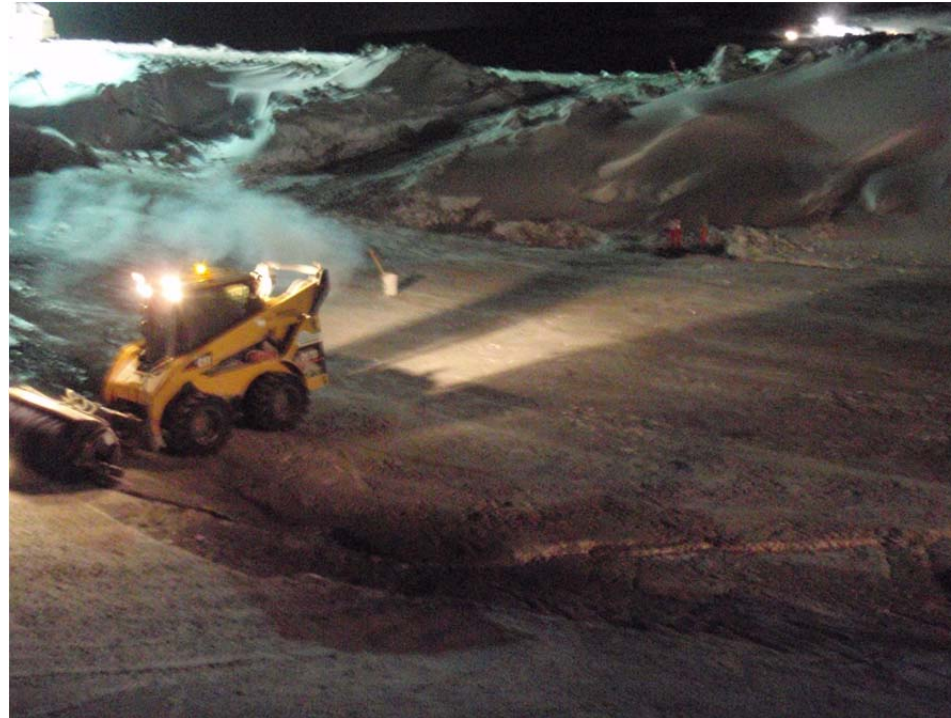
Photo 9: Bobcat (equipped with brush) cleaning the central key trench area before placement, ~ NW view.
