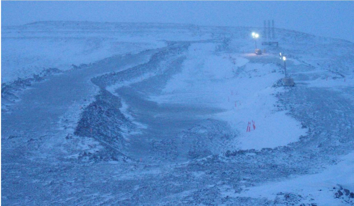
Photo 1: ~SWW view down key trench after ‘white out’ conditions were changed to Level 1 conditions in the am. Note the snow that has built up against the downstream bank of the key trench.
